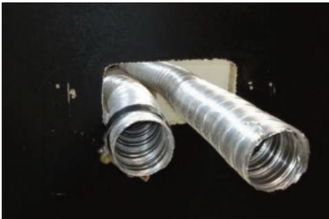
Cut flue exhaust tube (hot tube) to length (approximately flush with wall exit). Wall termination will sit against wall.
