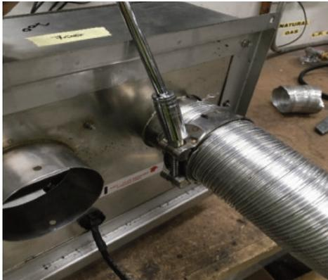
Slide flue onto connection spigot fully. Tighten clamp fully. Wipe excess silicon, visually check connection to ensure connection is fully sealed.
