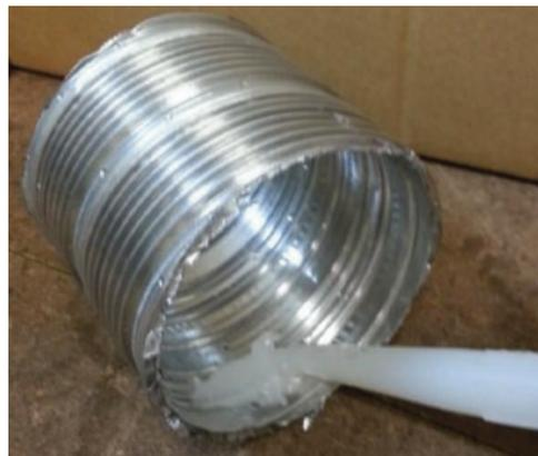
Apply an 8mm silicon bead fully around the inside of the flue end (heater connection end)
