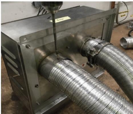
Feed air intake flue pipe through location spigot and fit retaining screw.
