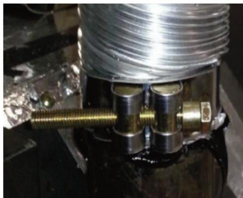
Slide flue onto connection spigot fully.
